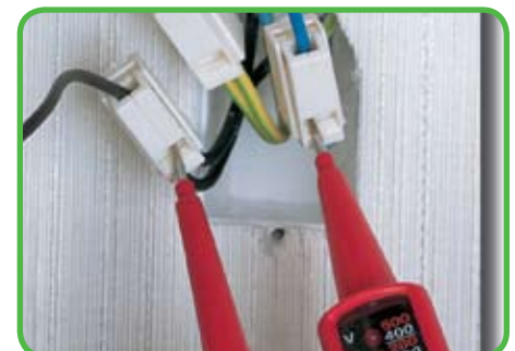
Testing through separate test slot
